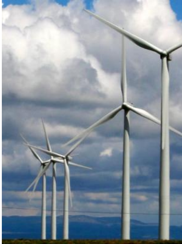
Figure 1.3 Typical wind turbines
